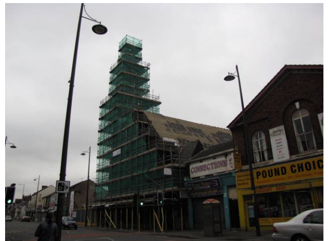
Site Development – July 2009
